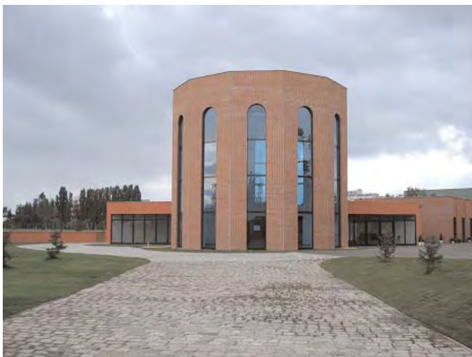
Figure 3: Front view of the new Islamic cemetery building in Vienna
